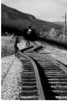
At each joint there must be a short gap ( $\approx 1/8''$ ) between the rail ends, to allow for longitudinal thermal expansion of the rails on hot days.
